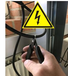
3.)Put the wire into the box and strip the ends of the wires and check if it has 4 or 6 cores
